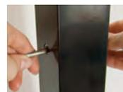
**Do not tension the cables completely until all the cables have been installed between the end posts.**
