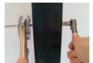
Go back and double check the tension of each cable, as tensions may change as each cable is continuously tightened.
